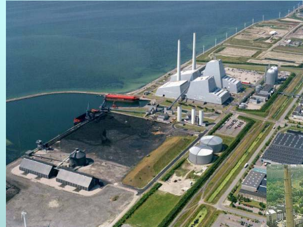
Avedore, Denmark – 70% wood + 30% gas/oil)
