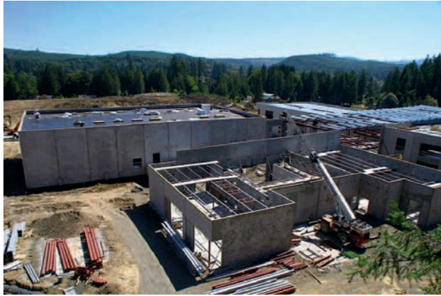
Progress is being made on the new LEED-certified school building, August, 2011.
