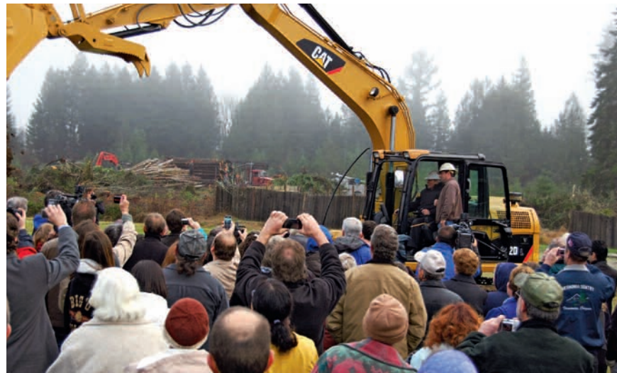
Former Oregon Governor Ted Kulongoski breaking ground at Vernonia's new school complex.
