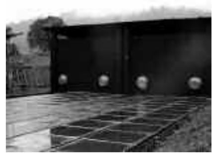
Solar Kiln, glass collector panels in front, kiln with exhaust fans.
